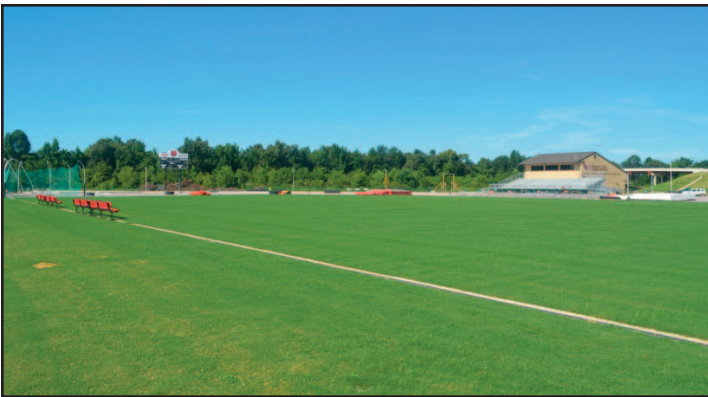
Track and Field/Women's Soccer Complex
